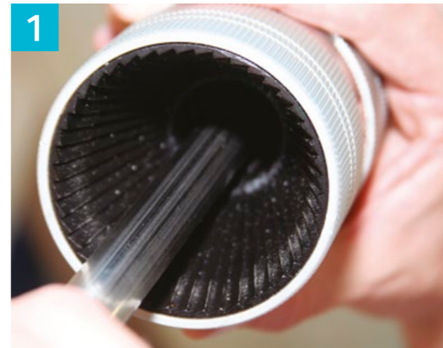
Cut and deburr pipe
