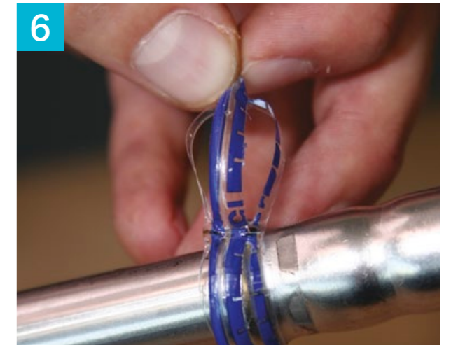
Remove pressing indicator
