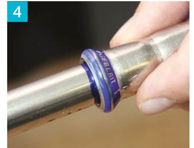
Insert pipe into fitting
